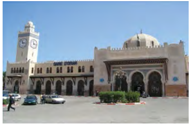
Station at Oran, Algeria. Photo: Wikipedia
