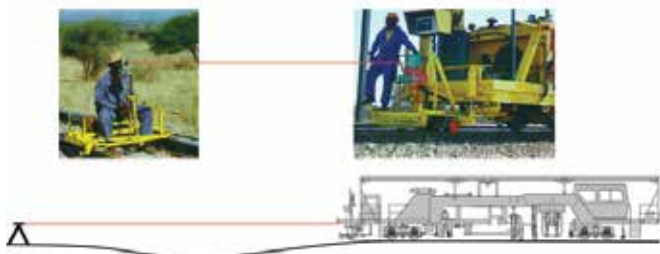
Figure 9: The use of optical (as illustrated) or laser equipment to permit removal of long wave defects
