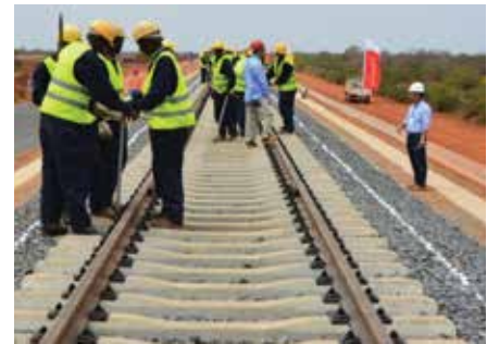
New standard gauge railway under construction in Kenya.
