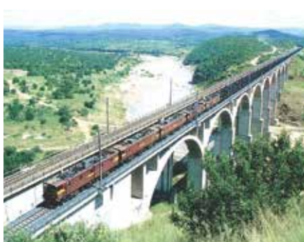
Heavy-haul: Umfolozi bridge. Photo: TFR.
