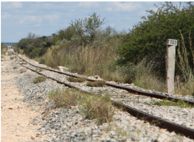
Condition of line before work was done
