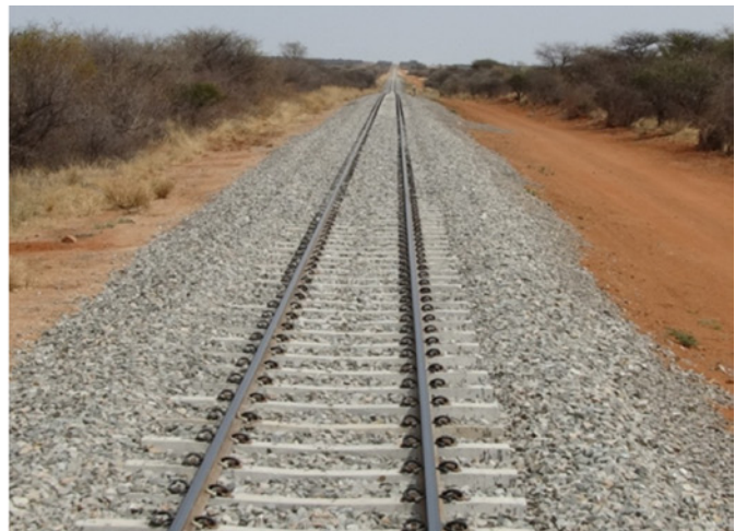
After completion of rehabilitation
