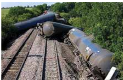
Derailment at Langworth
