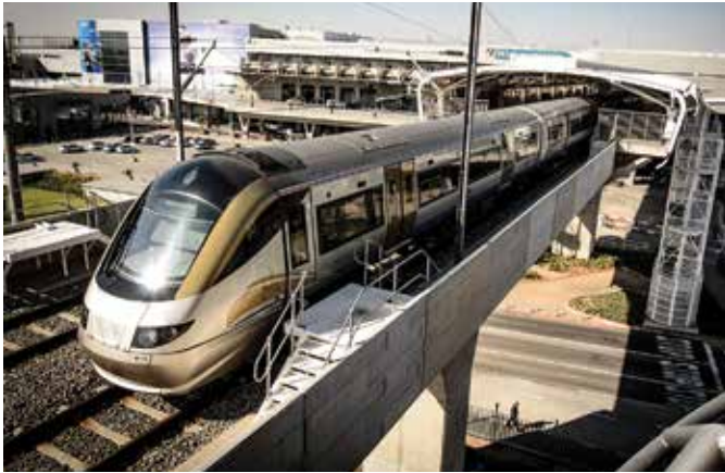
Gautrain airport station platforms: long enough for only two coaches
