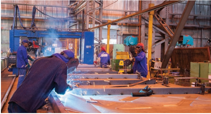
Transnet Engineering Bloemfontein wagon build. Photo Craig Dean
