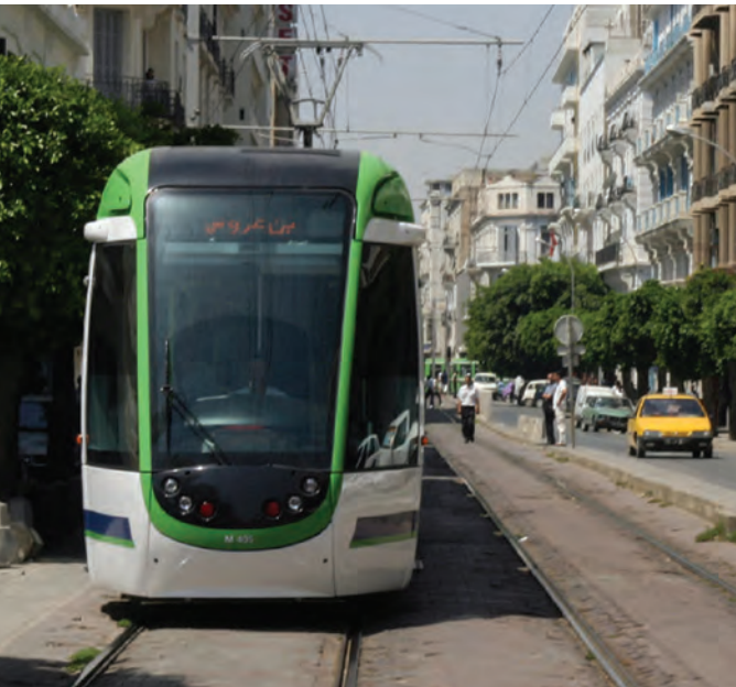
Citadis light rail in Tunis. Photo: Alstom.
